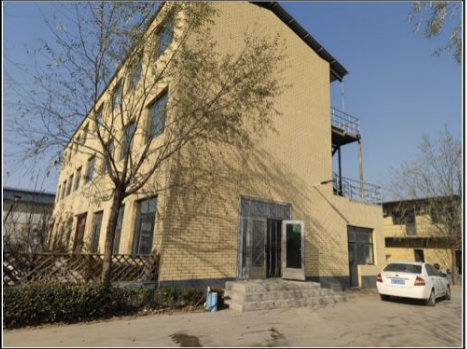
Block of offices
